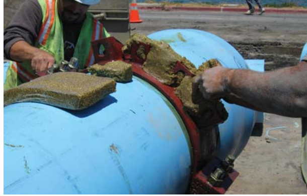
Coupling prepared with Prempaste and Prembond Mastic prior to Petrolatum Tape.
