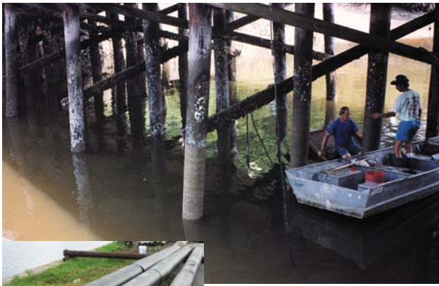
SeaShield Series 90 consists of Premtape Marine preventing marine borer destruction and an outcover for mechanical protection of tape.
