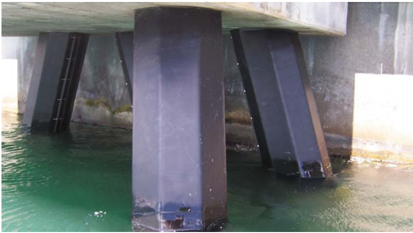
SeaShield Series 2000HD System was used to protect octagonal concrete bridge piles.
