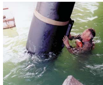
The components of the Series 2000HD System can be applied under water with minimal surface preparation.
