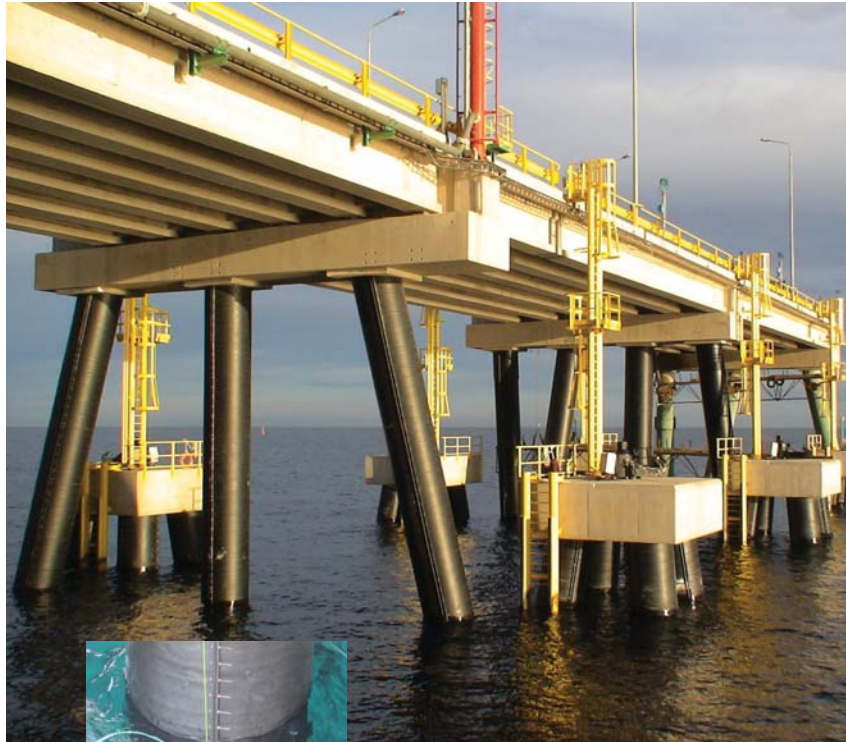
SeaShield Series 2000FD System designed to withstand the most aggressive environments.
