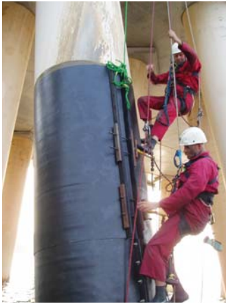
The SeaShield Series 2000FD System features a controlled application tensioning system.
