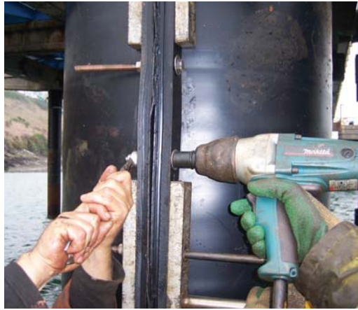
The SeaShield Series 2000FD System features a controlled application tensioning system.
