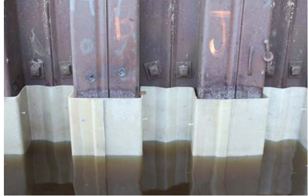
Structurally repaired timber piles with rebar, concrete and translucent SeaShield Fiber-Form fiberglass jackets. The jackets can be manufactured to be translucent or gel coated to a color.
