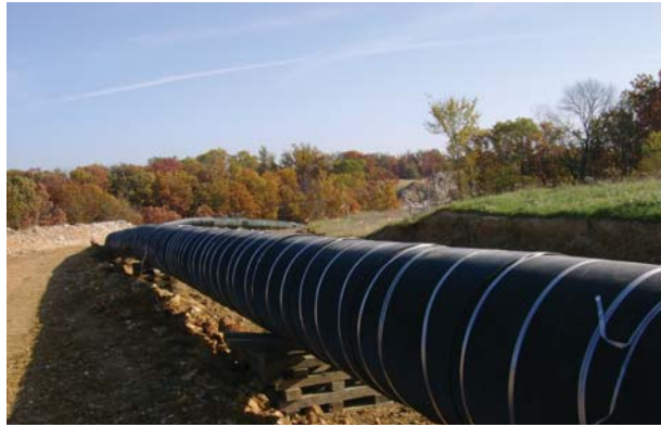
Premier Rock Shield HD is essential where pipelines are constructed through rocky terrain.
