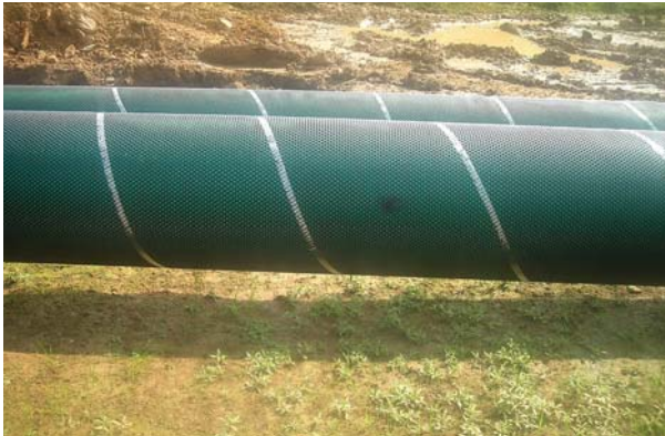
Premier Rock Shield SD can be easily applied and provides additional protection.
