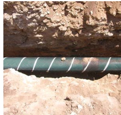
Premier Rock Shield SD in action, protecting the pipe coating.
