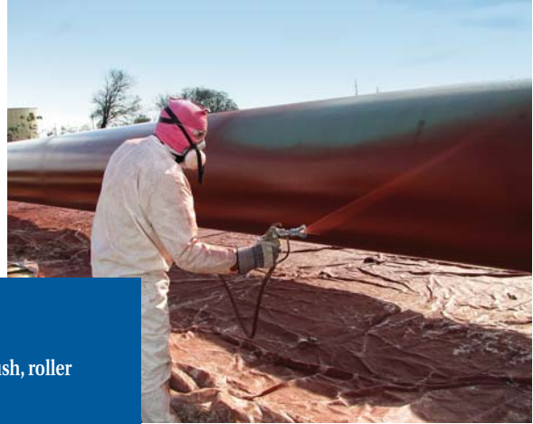
Protal ARO being sprayed applied.
