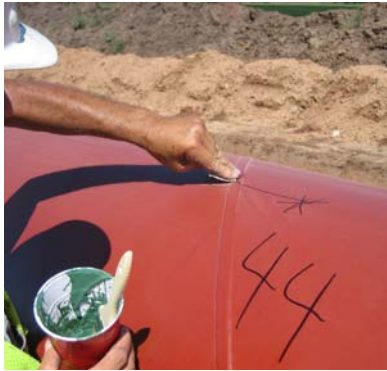
Protal 7125 being brush applied in arctic temperature conditions.
