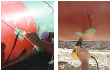
Protal Repair Cartridge application.
