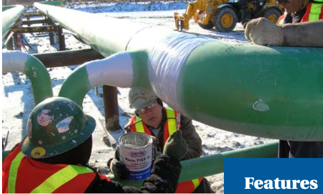
Protal 7125 being brush applied in arctic temperature conditions.
