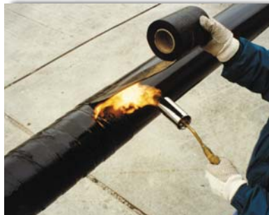
Pipeline rehabilitation and repair.
