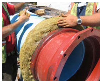
Minimal surface preparation (SSPC SP 2-3).
