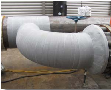
Cooling tower piping, tank bases and pipe under thermal insulation.
