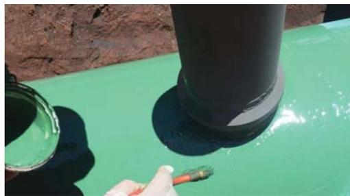
Protal 7200 being applied on the main line and on the difficult areas of the welded structure.
