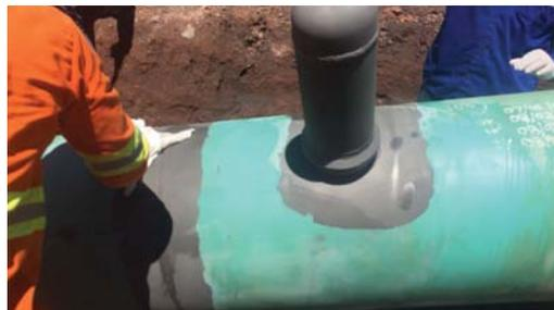
Contractor doing the surface preparation to SP-10 and anchor profile of 2.5-5 mil.
