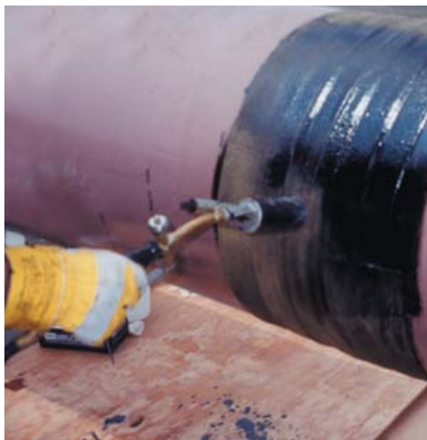
Application of heat on top of Premtherm Tape to seal overlaps.
