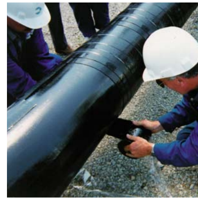
Application of Premcote 150R.
